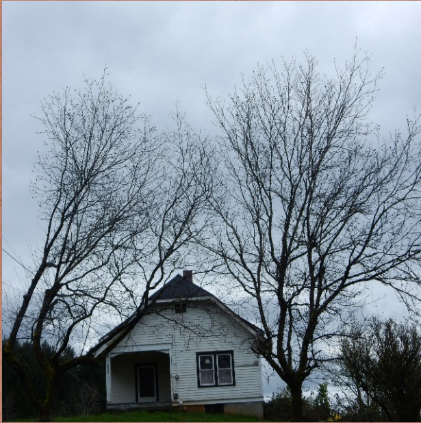
WILSON SCHOOLHOUSE 53500 NW Wilson School Road Forest Grove, Oregon STATUS: Spooky
