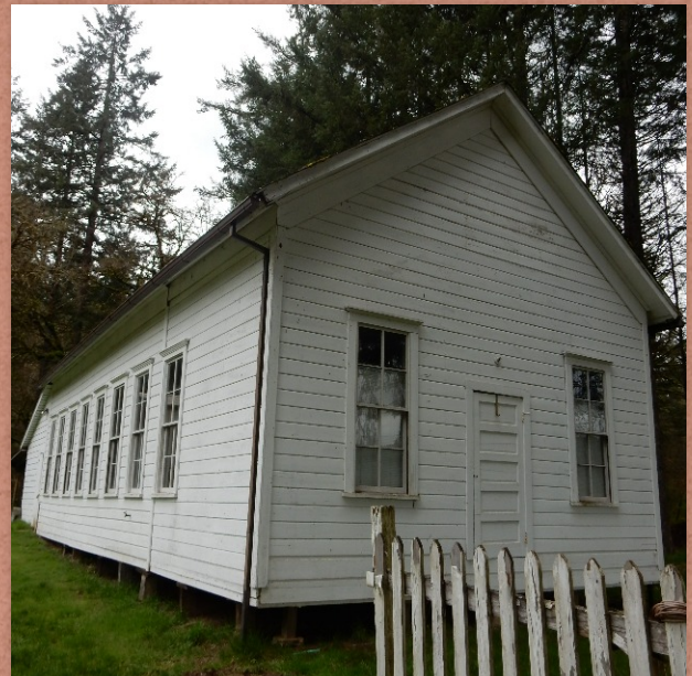
MOUNTAINDALE SCHOOLHOUSE 15915 NW Dairy Creek Rd North Plains, Oregon STATUS: Well-Tended
