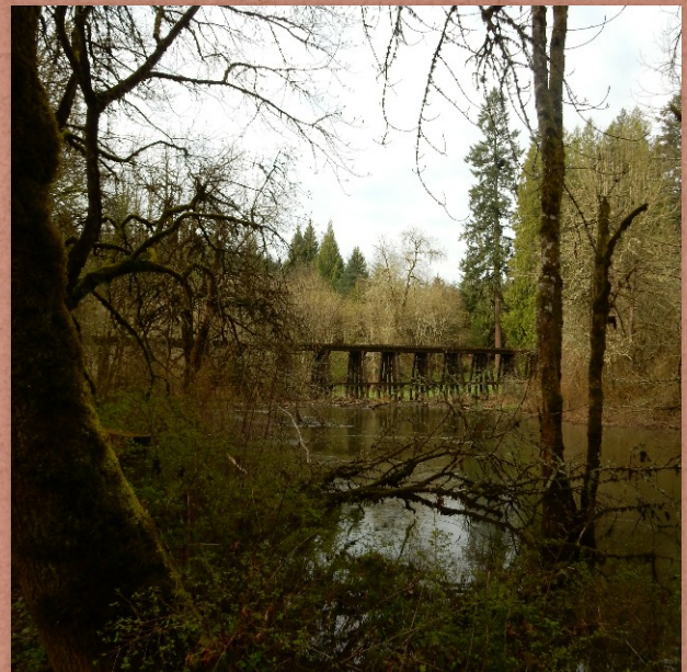
DAIRY CREEK TRAIN TRESTLE 515 SW 17th Ave Hillsboro, Oregon
