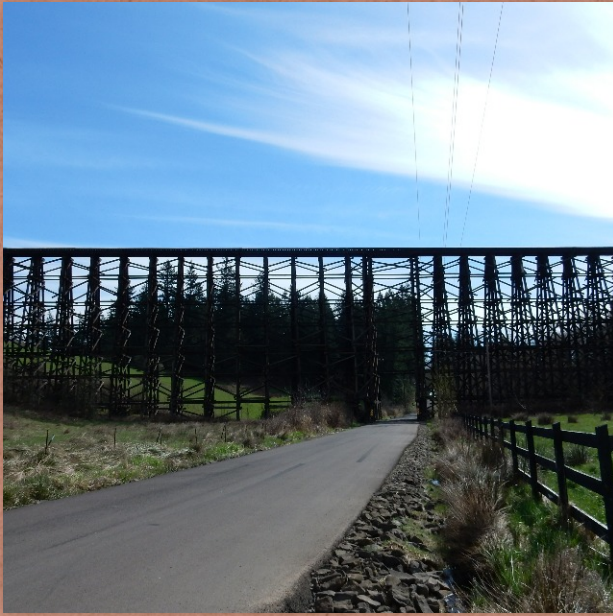
HOLCOMB CREEK TRESTLE BRIDGE 10500 NW Dick Rd Hillsboro, Oregon
