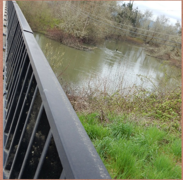
SCHOLLS FERRY BRIDGE 23545 SW Scholls Ferry Rd Hillsboro, Oregon
